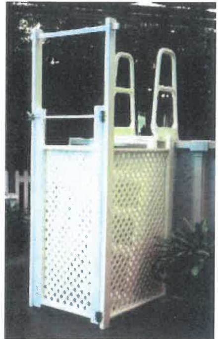
Fence around ladder area
