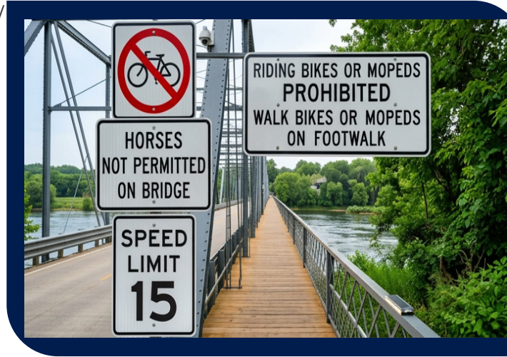
Obey the posted regulations on bridges.
